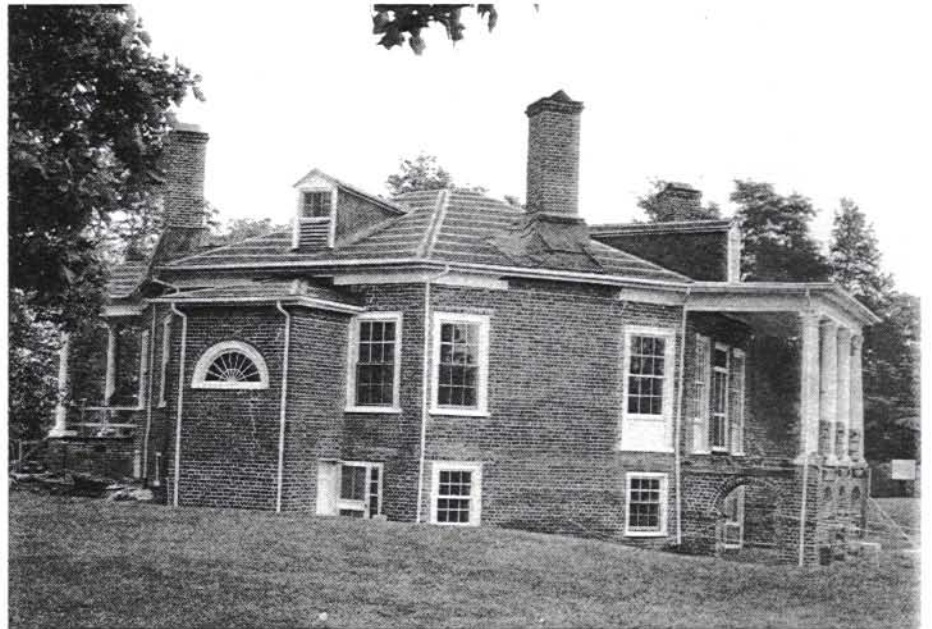
Fig. 9. Poplar Forest showing the 1945 changes with reopened window openings. Windows were lowered about 1' in the wall during the 1846 rebuilding and the triple sash windows of the parlor lowered and altered with jib doors. Photograph by author.
