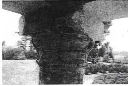
Fig. 7. Tuscan capital stripped of its rendering. Photograph by author.
