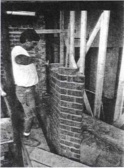
Fig. 10. Restoration mason Henry Cersley restoring a window opening. Photograph by author.
