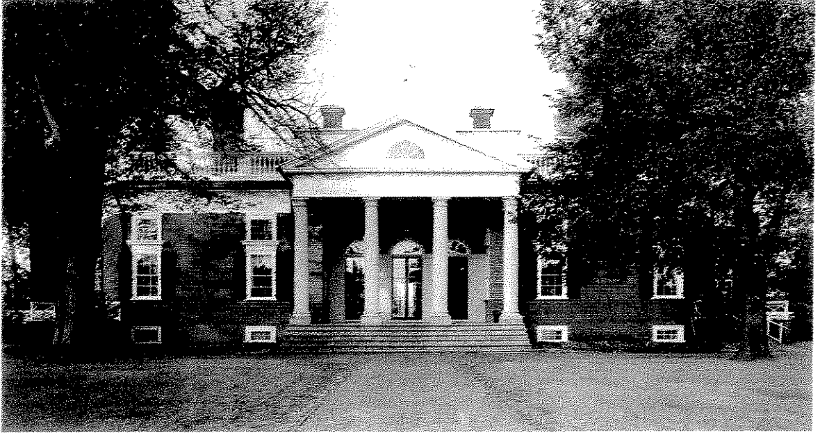
FIGURE 50: Front elevation of Monticello. Note the second story windows joining the tops of the first story windows, lending the appearance of a single story elevation. This "modern" innovation Jefferson brought back from France.
