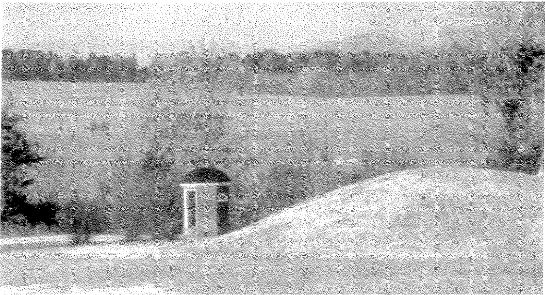
FIGURE 4: Close-up of west mound and octagonal privy, both original landscape elements.
