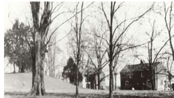
Above: East mound, north and south tenant houses, looking northeast
