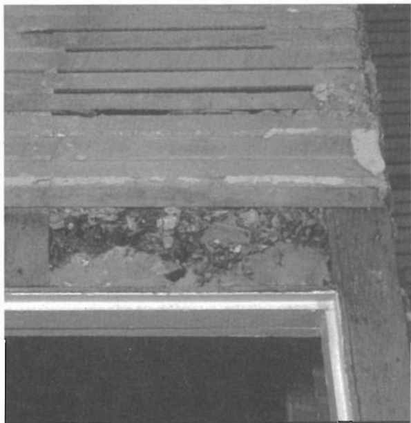
FIG 11.4 The largest nest at Poplar Forest was located vertically in the stud walls of an enclosed staircase from the middle room and spread horizontally between the floor boards of the attic above. Photograph by the author.
