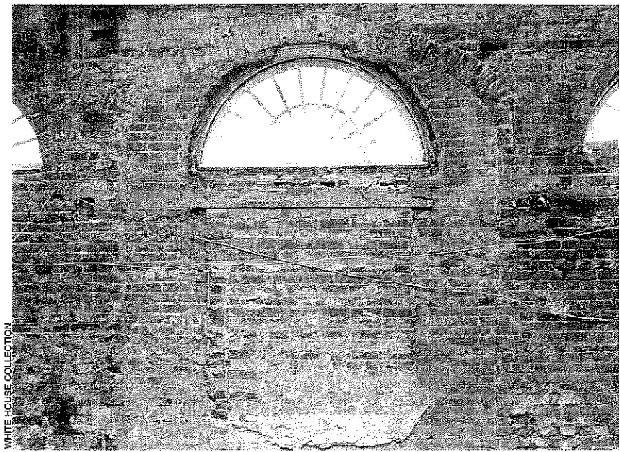
24. Top: In this 1969 photograph, the eighth window bay (from the east) of the west wing shows a much larger opening that has been filled.
